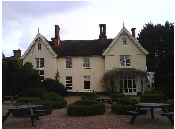
Photo above shows the Cornwallis Hotel in Brome
