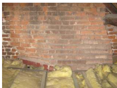
Steel beam supporting chimney breast in loft
