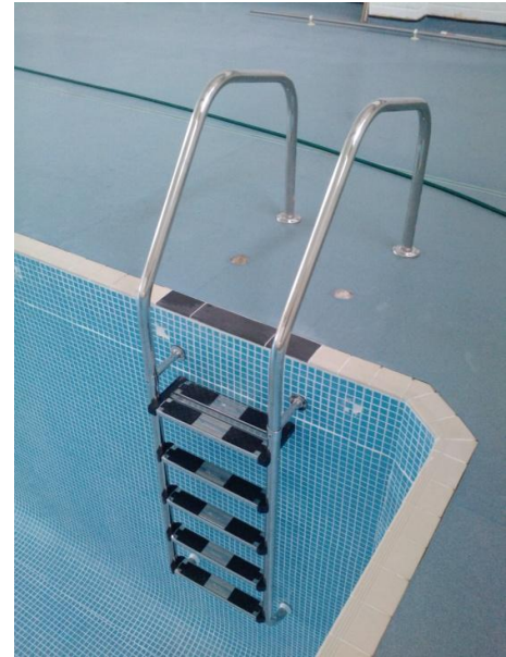
Aug 2009 Cleaning and re-grouting of Swimming Pool Mosaic tiles. Including new pool steps to current regulations.
